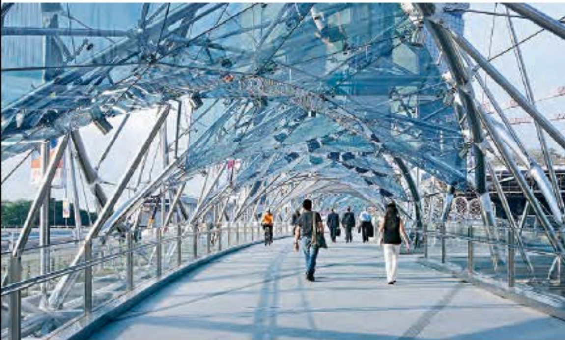
Beneath the stainless steel curves, pedestrians are protected from the sun and tropical rain by shade canopies. Photo: Financial Dynamics/Christopher Frederick Jones
