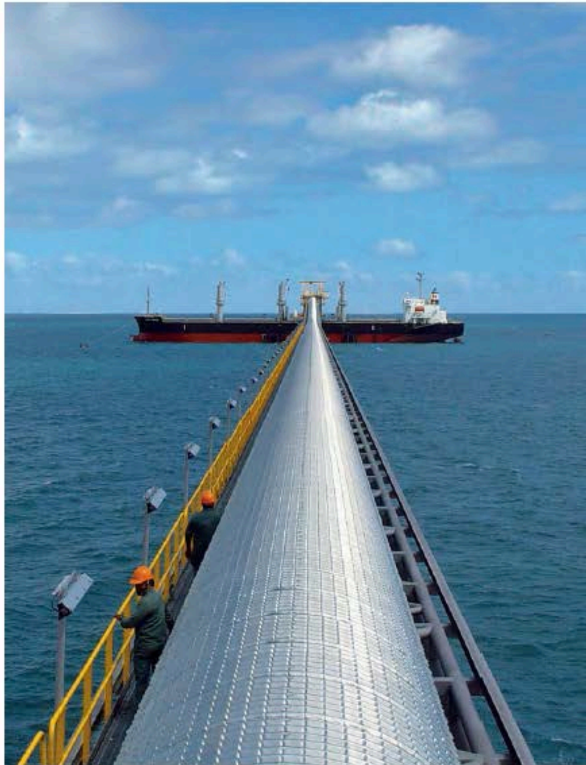
Conveyor for nickel ore in New Caledonia, stretching 1.2 km (0.75 miles) into the sea (total length: 1.8 km, or 1.13 miles). Subject to a strongly saline atmosphere, to shocks and to jolts, the quality of its lubrication is essential for its reliability. Photo: Eramet-SLN.
