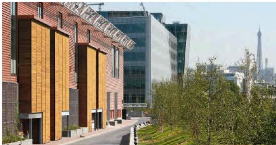
View of the waste plant façade facing the Seine. Photo: SYCTOM
