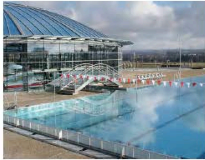
The Bellerive-sur-Allier swimming pool, Vichy. It was the first Olympic-size swimming pool in France ever to be built of stainless steel. Photo: Jacques Rougerie.
