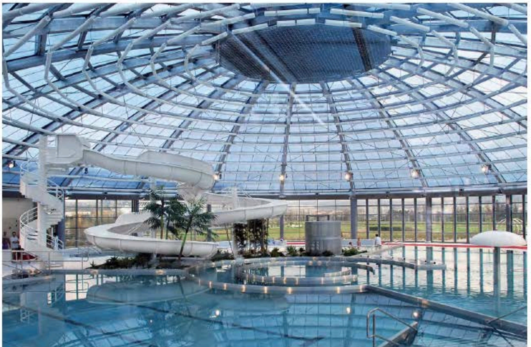
The Bellerive-sur-Allier swimming pool, Vichy. The stainless steel lining allows the designer to create complex shapes that are difficult to realize with other building materials. Photo: Jacques Rougerie.
