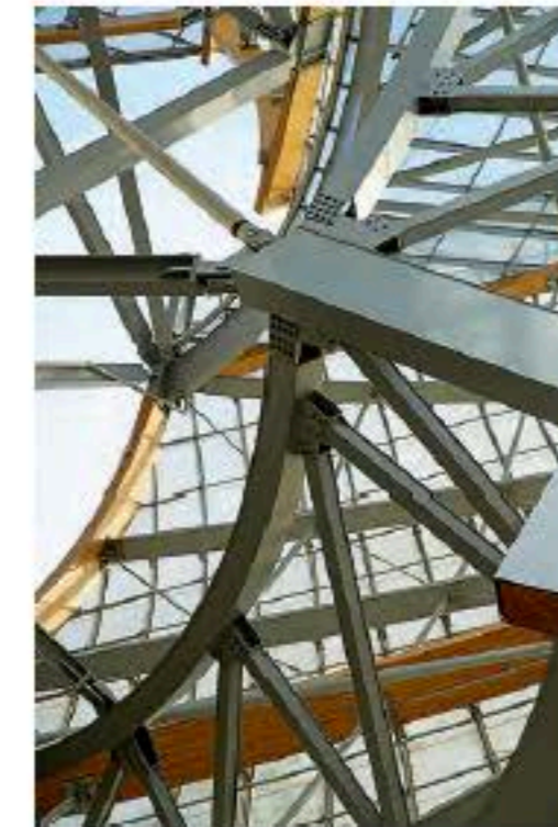
The roof support structure is made of wood, steel and duplex stainless steel components. © Eiffage
